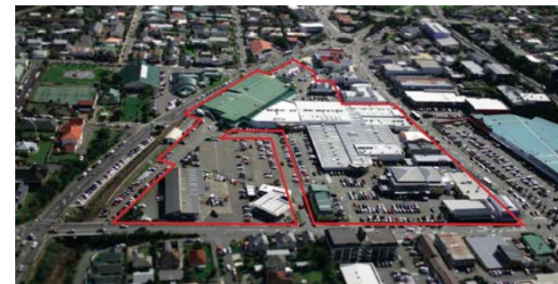
Johnsonville Shopping Centre, Wellington
